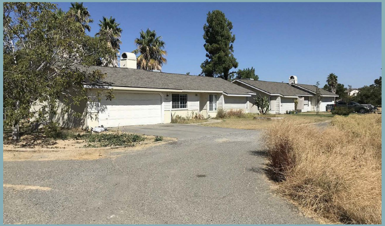
Figure 4.1-8 Existing On-Site View of Duplexes in Central Portion of Project Site
